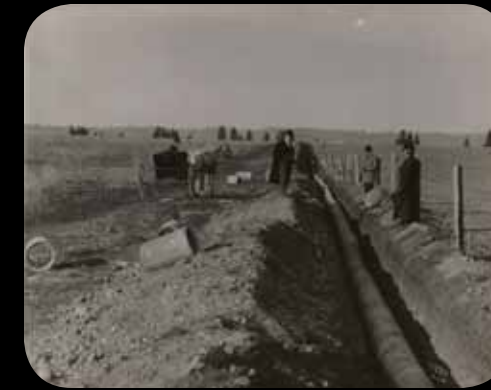
Laying irrigation pipes, 1908
