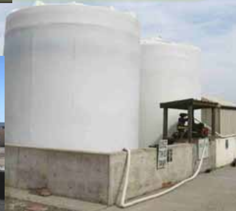
Concrete containment
