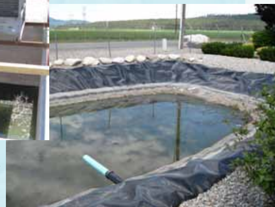
Passive wastewater evaporation pond
