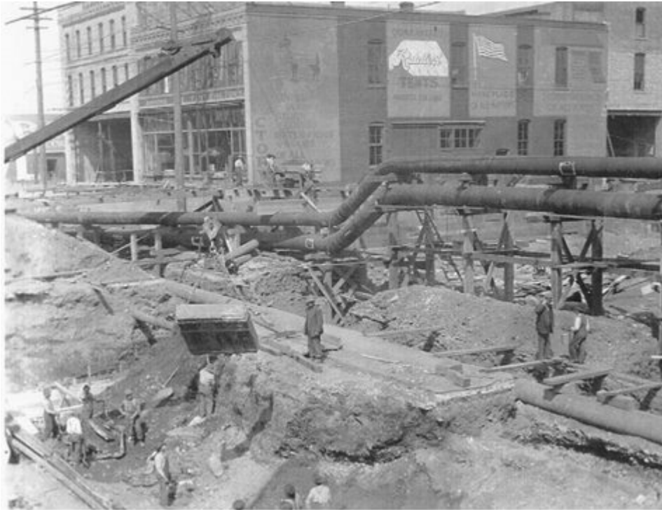
Main relocation for railroad grade separation near Division and Trent (now Spokane Falls Boulevard) in 1911.
