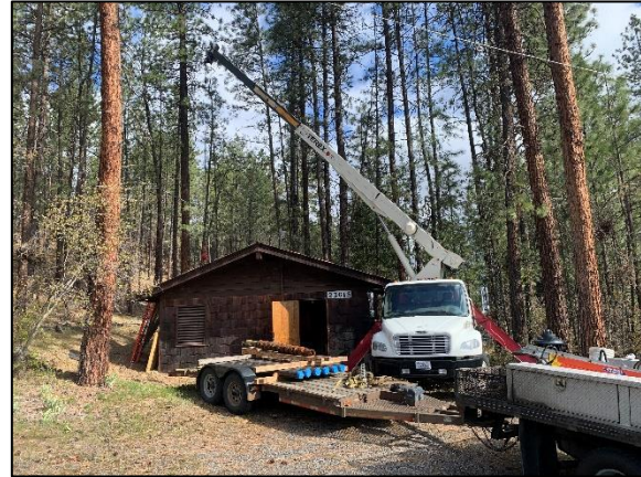
Crane Setting New Pump and Motor in Place
