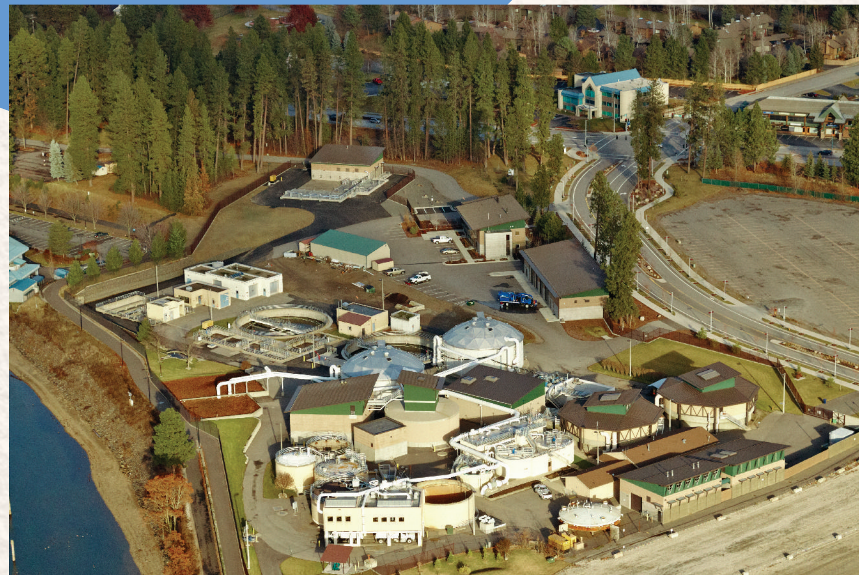
WASTEWATER PLANT NOW Adding a tertiary removal process to the wastewater treatment plant has helped the quality of water in the Spokane River and neighboring areas. Removing phosphorus means cleaner water, healthier environment, and a happier community.
