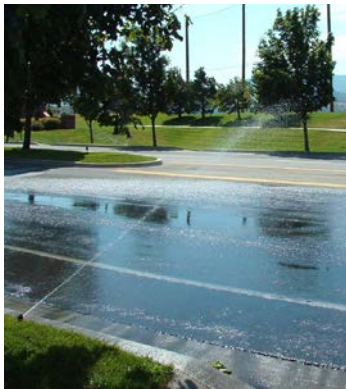
Sprinkler systems left unmaintained can cause runoff and damage hardscapes.
