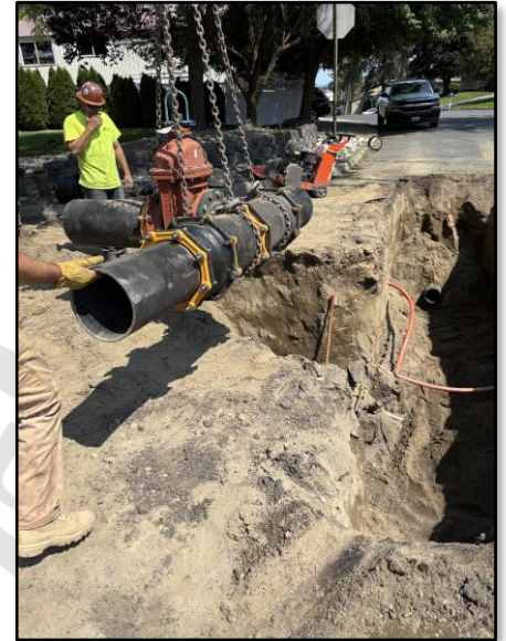
Employees from Sonray Enterprises Installing a 12" Tee on Cascade Way
