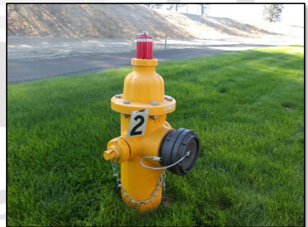
Locked Hydrant to Prevent Misuse
